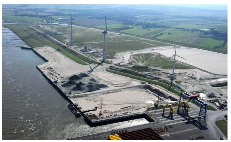
The order for the construction of the offshore LP 9 in Cuxhaven was generated by a joint venture of F+Z Baugesellschaft (today Depenbrock Ingenieurwasserbau), Josef Möbius, Tiefbau GmbH Unterweser and Heinrich Hirdes via a secondary bid with optimized finger pier and sheet pile wall construction. Execution took place between March 2010 and December 2012.
