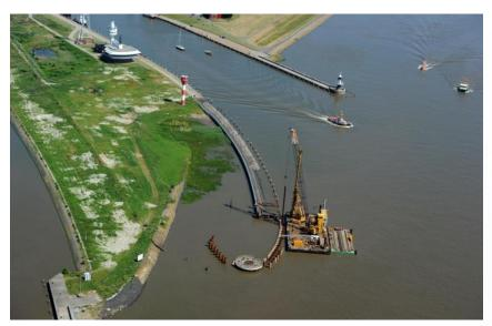
The lighthouse "Mole" will be moved about 50 m westwards. The existing pierhead will damaged on a length of about 25 m and a 75 m long pier construction will be build.
