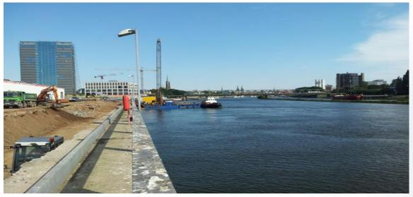
Construction of a new Quay wall in front of an existing structure in the vicinity of "Weserbahnhof 1" in the City of Bremen with a length of 356 m, consisting of a combined steel sheet pile wall, anchored by inclined micropiles including equipment, super-structure as well as flood protection wall, reinforced concrete wall and steel wall.
