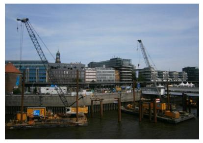
The joint venture under the technical management of F+Z Baugesellschaft (50%) was commissioned with the new construction of a 310 m long flood control wall with an existing promenade and parking garage behind.
