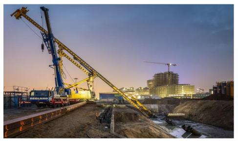
In Hamburg Hafencity in the area of the former Grasbrook, a shopping centre, a cruise terminal, two hotels and various entertainment facilities are under construction. The site is characterised by its former use of Hamburg's gas works. Old building structures like foundations and pile remains are to be expected.
