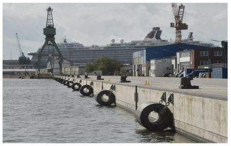
The construction measure put out to tender here comprises the renovation of the western quay in Kaiserhafen III and the construction of a jetty for berths for the ships and barges of bremenports' maintenance dredging and work ships. The work is being carried out in a joint venture with Aug. Prien.
