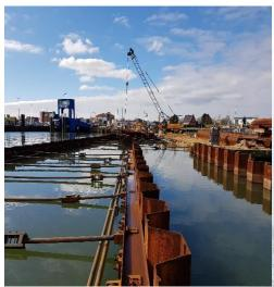
Upgrading of ferry pier 1 in the port of Wyk auf Föhr. The new construction will enable the separation of car and pedestrian traffic. Rehabilitation of the old jetty, some of which is in a state of disrepair, by means of sheet piling with tiebacks consisting of round steel anchors and grouted piles. Reinforcement of the transverse breakwater. Island construction site complex work preparation. Driving of the coated dolphins with attachments welded on one side under high demands on accuracy.
