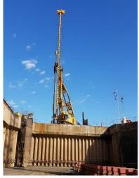
An existing dry dock measuring 195m x 35m (LxW) is to be extended by 7m on behalf of Varvsudden Industrial Park. The width of the extension is 11m.
